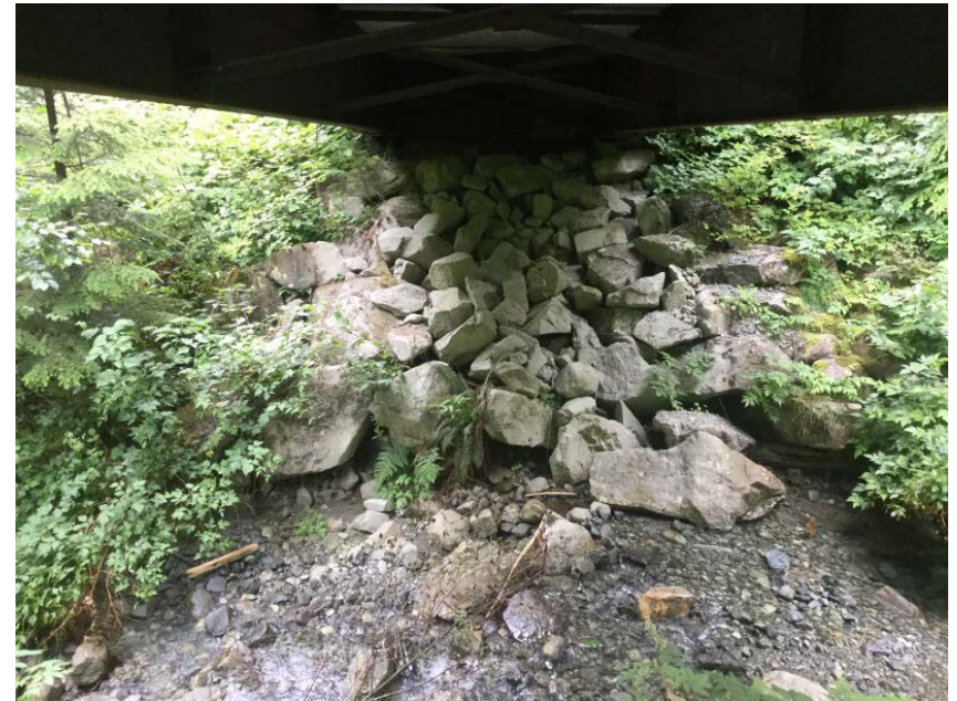
Right Bank Abutment when facing downstream
