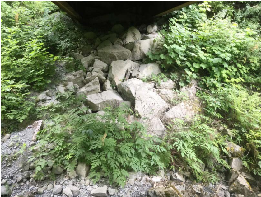
Left Bank Abutment when facing downstream
